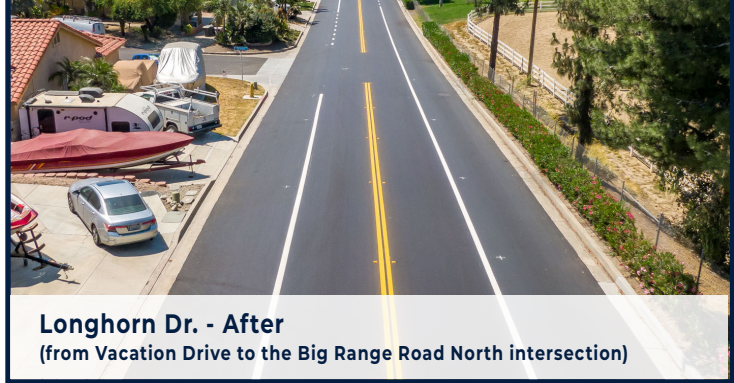
Longhorn Dr. - After (from Vacation Drive to the Big Range Road North intersection)
